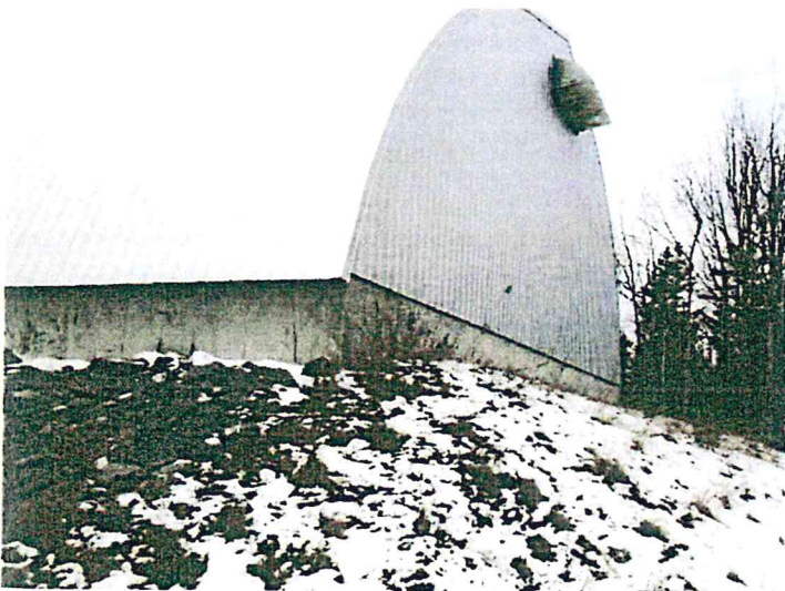
Easterly portion of the site
