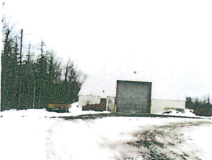
Centrally located looking east
