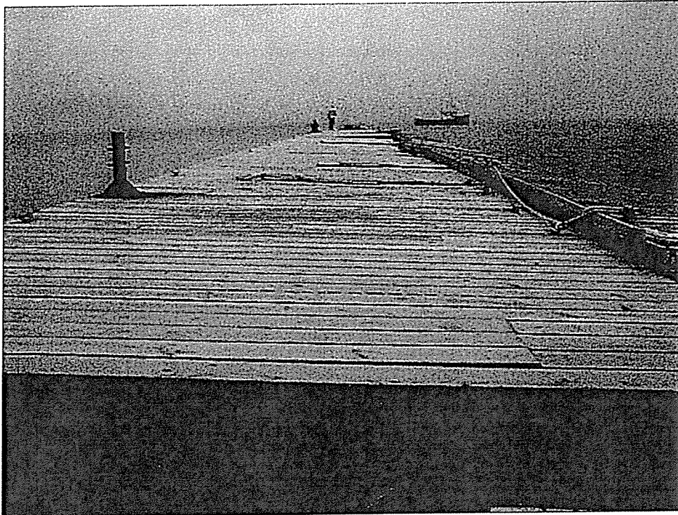
Photo 5 – Top of floating breakwater/wave attenuator. Note new decking.
