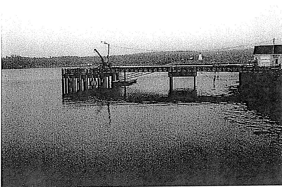
Photo 4 – Permanent concrete town pier.
